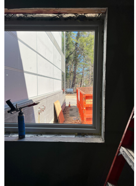
Above: Window installation
